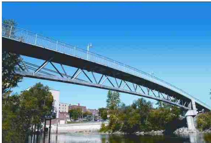
Figure 1.2. Sherbrooke prefabricated pedestrian bridge, 1997, Canada. (ACI 239 C 2015)
